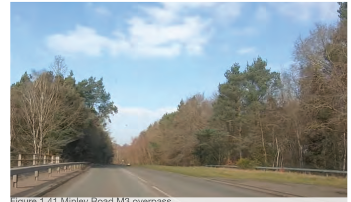
Figure 1.41 Minley Road M3 overpass
